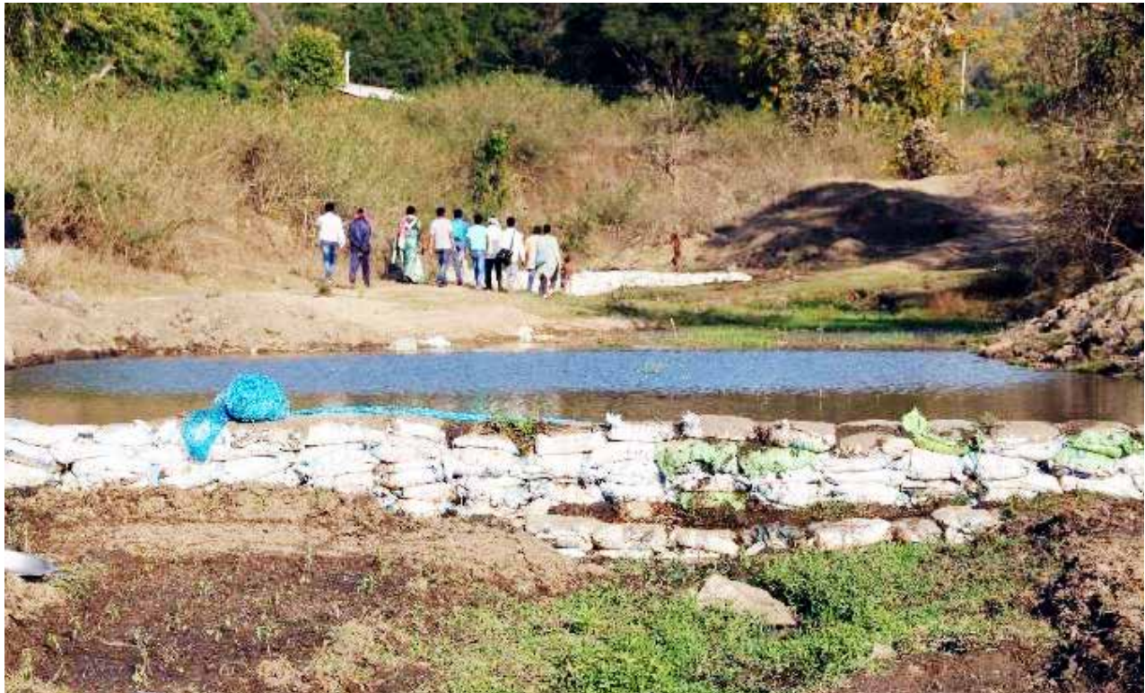
Bori bandha (temporary bund) made by community for water conservation
